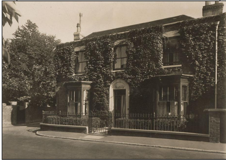
This house (191 Canterbury Road) is shown as the 'Charity School' on the 1840 Tithe Map
